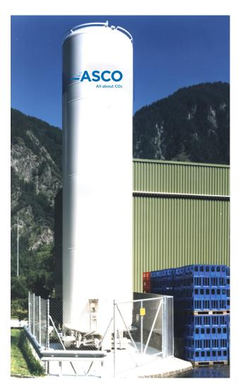
ASCO CO<sub>2</sub> Storage Tanks include a high quality perlite vacuum insulation and are supplied complete with all pipework, valves, safety devices, liquid level indicator, pressure gauge, automatic pressure build up and pressure reducing systems allowing fast and easy installation on site.
