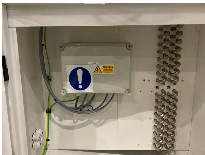
Terminal box for external control cabinet
