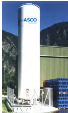
Vertical CO 2 storage tank
