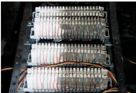
Cleaning of a switch board of a national Telecommunication Company. In this way short circuits can be avoided.
