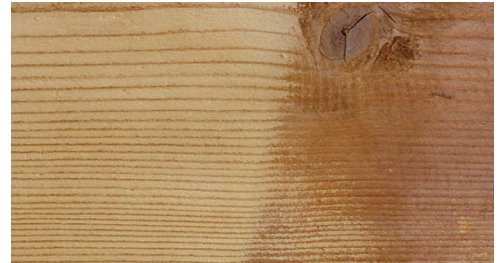
Wooden façade before and after cleaning
