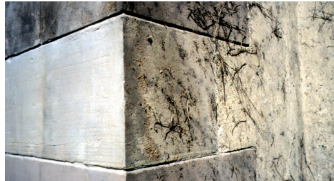
Stonewall before and after cleaning
