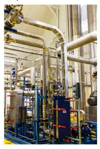
The shown process unit consists of various pumps and heat exchangers and is responsible for heating or cooling of the  $CO_2$  gas and the wash solution.
