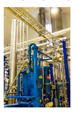
The CO<sub>2</sub> compressor compacts the CO<sub>2</sub> gas to a pressure of 16 to 20 bar.
