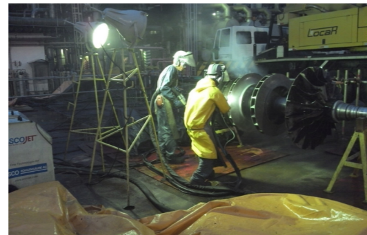
Cleaning of gas turbines
